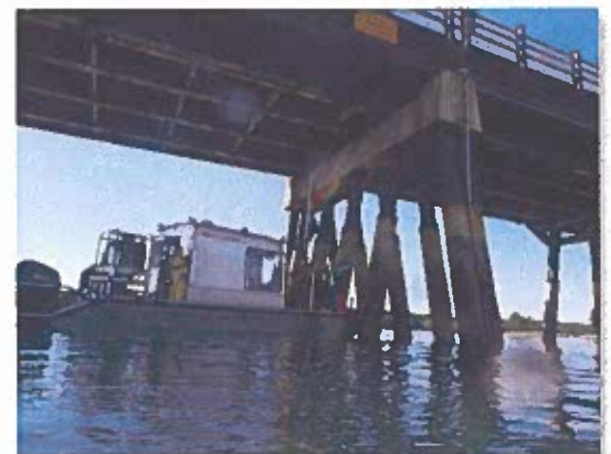
Bridge substructure inspections
