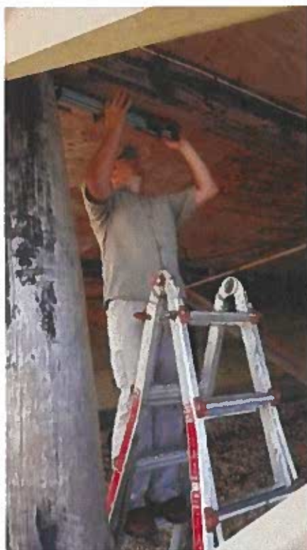
Resistograph PD Series field deployment — resistance drilling of structural timber elements for relative density profiling and internal condition assessment.
