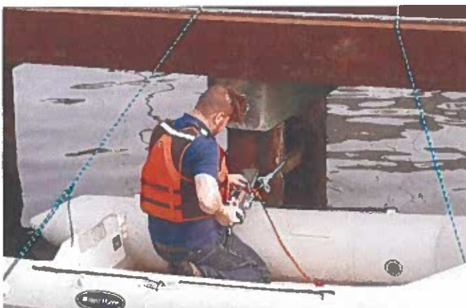
Photos of Engineer Dive Inspector, Robert Provencher using the resistance drill at a recent site inspection
