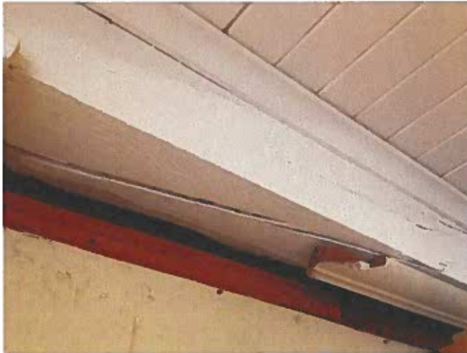
Steep slope of grain revealed by a large split — this timber was classified non-structural with a partial in-situ failure.
