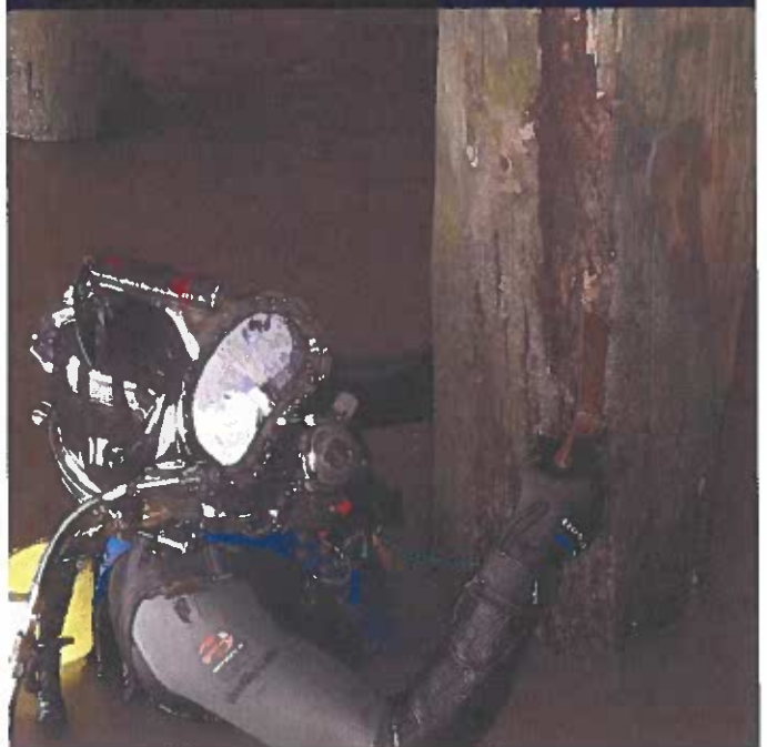
John Gaul, PE - ADCI-Certified Diving Supervisor and NC PE Inspecting Timber Piles at MOTCO Facility
