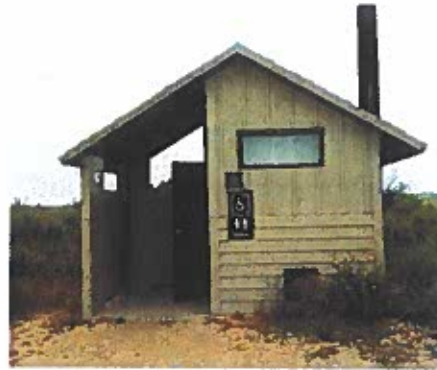
Example of waterless restroom
