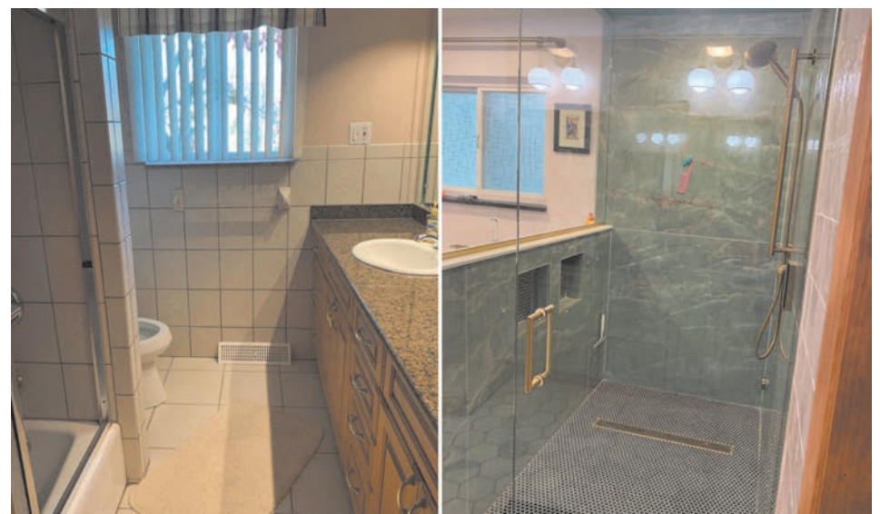
Nancy George's bathroom before and after remodeling.
