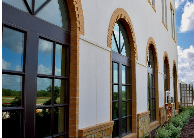
2014 GOLDEN TROWEL AWARD FIRST PLACE, BLOCK CATEGORY SAN ANTONIO MASONRY CONTRACTORS ASSOCIATION
