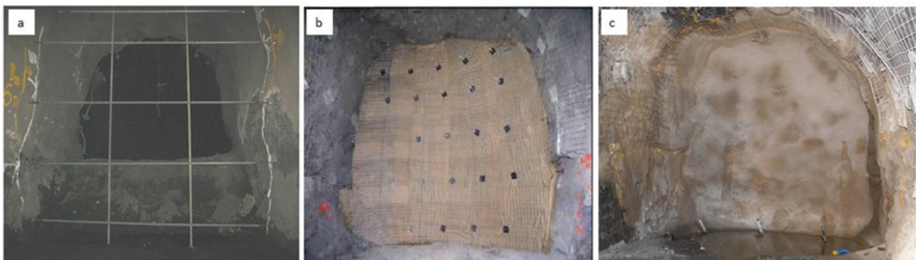
FIG 2 – Formwork and steps of construction of fibrecrete bulkheads (a) pre-fabricated arch placement (b) placement of the mesh and hessian over the arch (c) sprayed fibrecrete.
