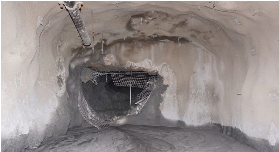
FIG 3 – Drive side of failed paste wall with fill pipe through wall (after Department of Mines, 2020).
