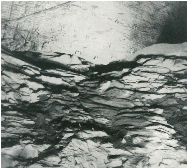
Figure 23: Rock fracture in floor during cavern excavation (Endersbee and Hofto, 1963; Hydro Tasmania Archive)
