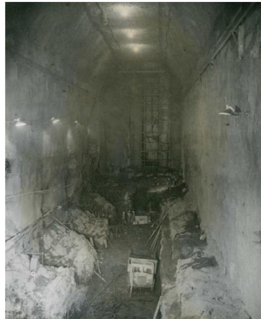
Figure 24: Condition of final cavern excavation (Hydro Tasmania Archive)
