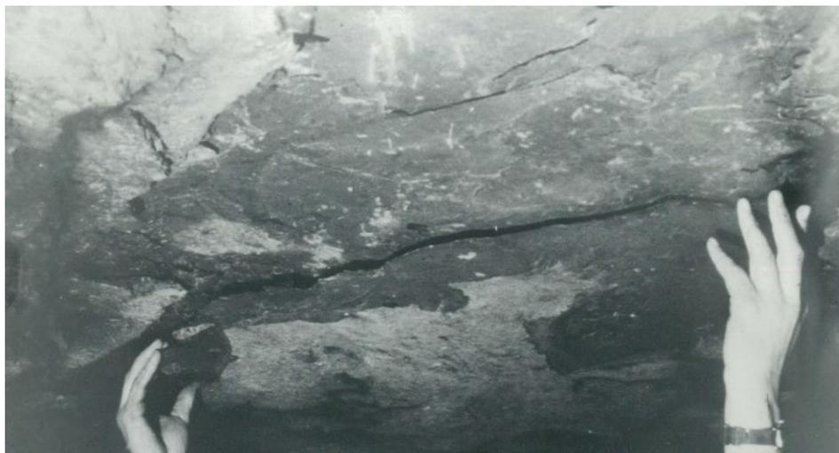
Figure 13: Slabbing in the roof of the unsupported crown drive (Endersbee and Hofto, 1963)
