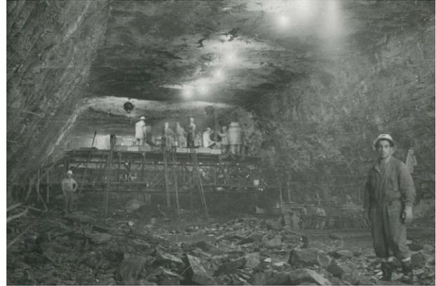
**Figure 18: Condition of top heading during late stages of excavation (Hydro Tasmania Archive)**
