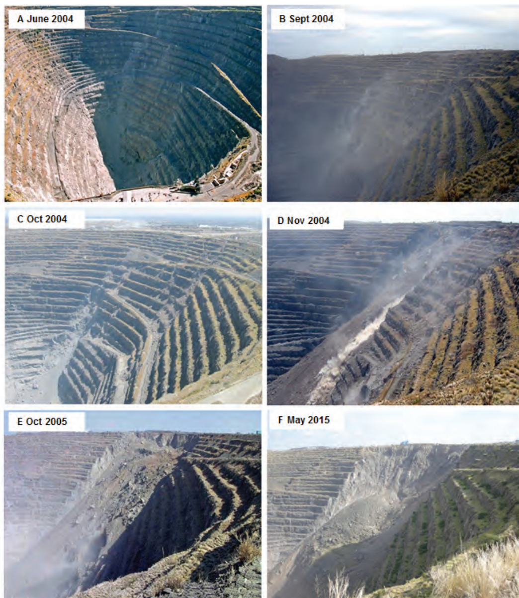
FIG 2 – Evolution of the north wall failure (looking north-west).
