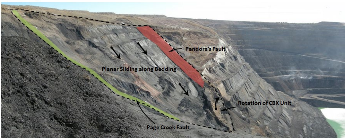
Figure 3 Conceptual model of the west wall progressive movement mechanism presented on views looking west (above) and north (below)
