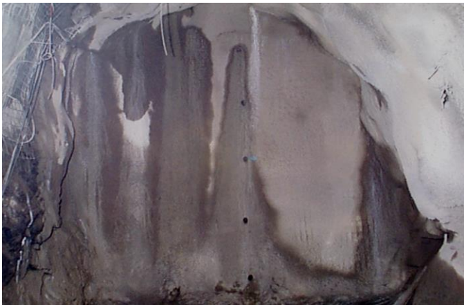
Fig. 1. Typical sprayed shotcrete/fibrecrete paste bulkhead.
