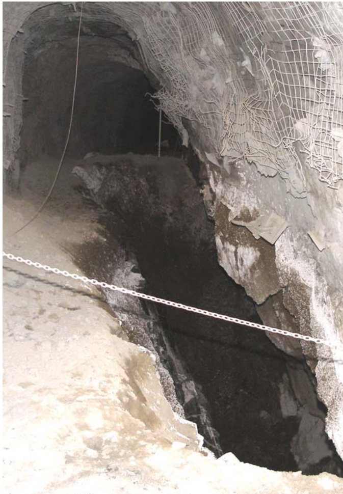
Fig. 2. Vertical paste fill exposure at the Raleigh Mine.
