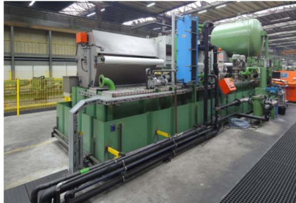
Mill Coolant Handling
