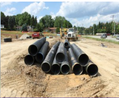
Storm Water Management & Permitting
