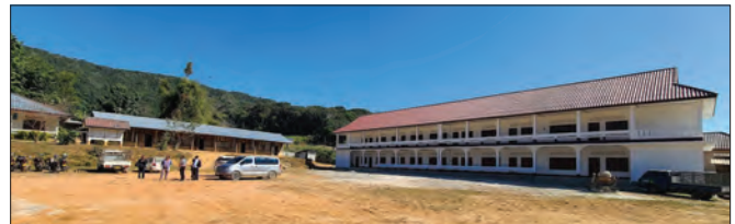
Nearly complete new Yun Xay classroom building above at right. Shed to the left is full of electric motorcycles. They also found such bike sheds in the more wealthy, well-established schools near Phonsavan. The city folks, and those living along the main routes, seem to be doing much better than in remote villages.
