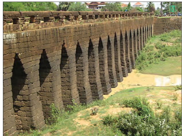
Above, the twenty corbeled stone arches of Spean Praptos date from the time that nearby Angkor Wat was built, nearly one thousand years ago.
