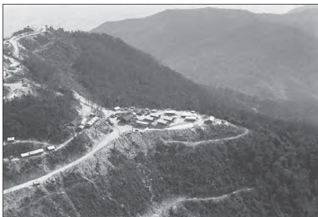
View of "Monkey Mountain," an aerial surveillance site very close to Danang Air Force Base along the coast of Vietnam, South of the DMZ.
