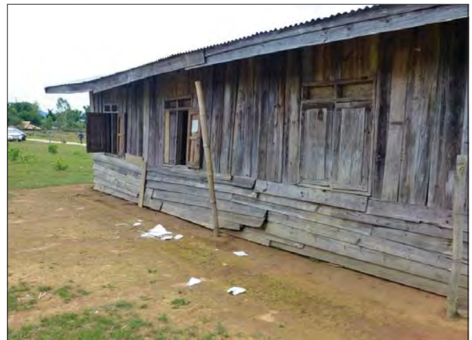
The deteriorating school at Ban Nong.
