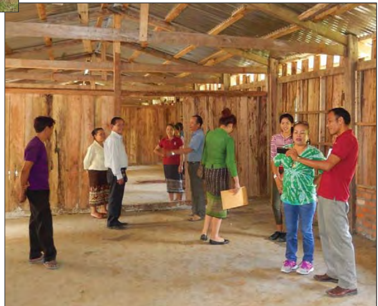
Above, the TLCB/Lao school team inspecting a new roof and floor funded by member donations to the TLCB Assistance.
