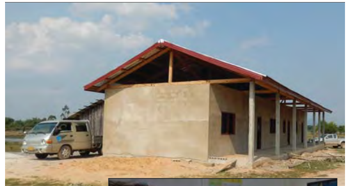
Above, Ban Nong School is nearly complete
