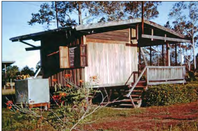
Phil's Thai government-provided little house was "palatial." Note the galvanized steel water tank; contents were carefully conserved during the long dry season.
