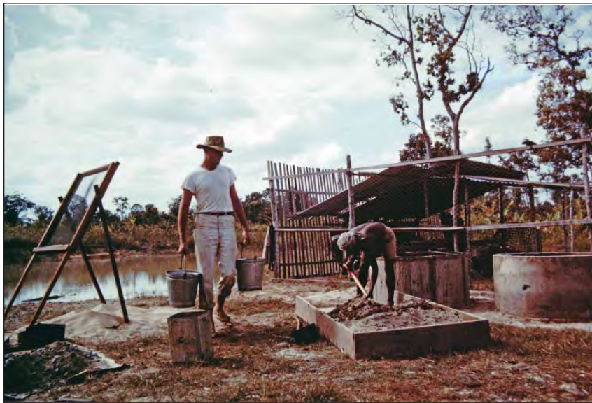
Left, hauling water and mixing concrete to pour well casings. Three hand-dug wells were completed during Phil's tour.
