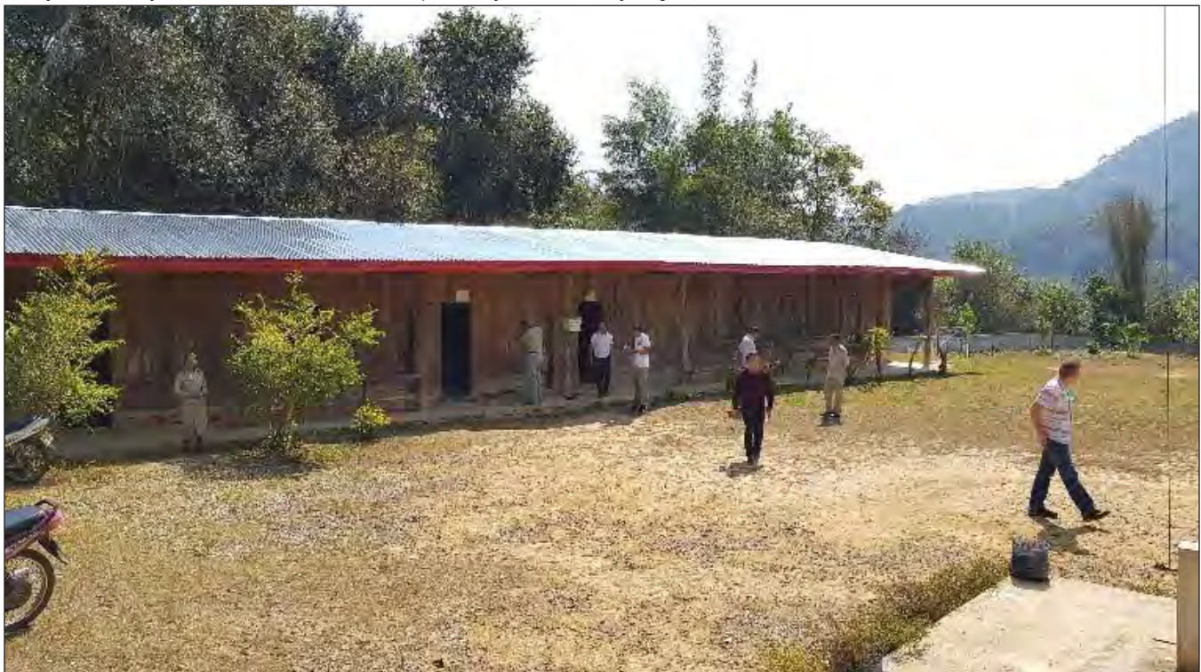
Ban Sy Chom Primary School with new roof sheets. Photos provided by the author and by Vaughan Smith.
