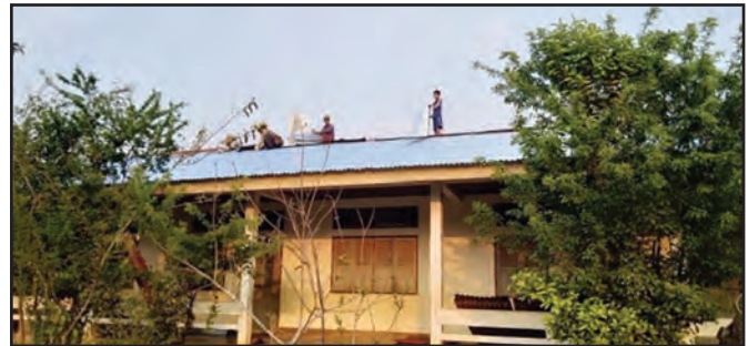
Above, Sy Vieng Kham Primary School, with new replacement roof sheets. Below, Kitchen roof sheets replaced also.
