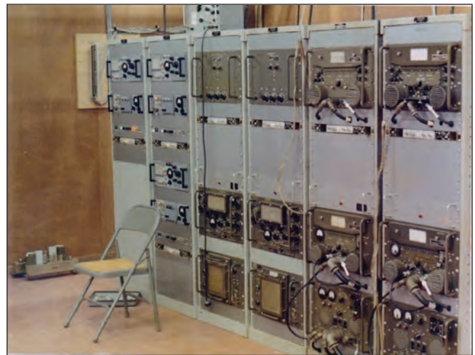
UHF transmitter/receiver installation at NKP.
