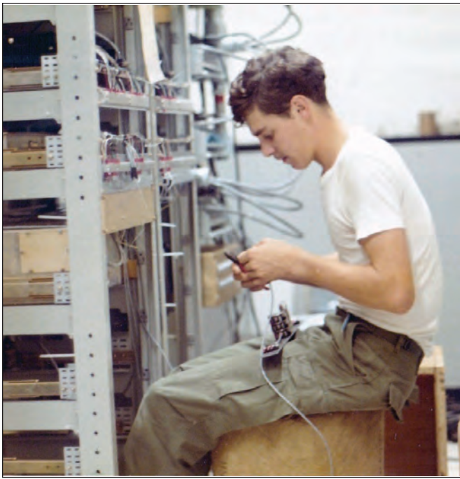
A1C Vettel installing UHF transmitters at Udorn.
