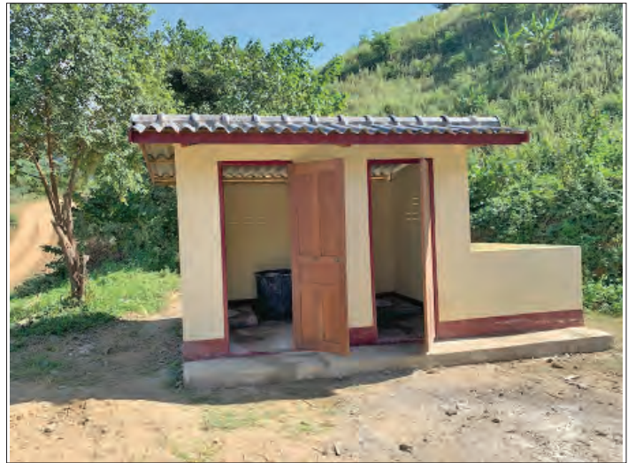
New toilet at SopOr School, thanks to the TLC Brotherhood Assistance Program! All photos courtesy of Paul Carter and Vaughan Smith.
