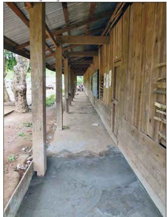
Long Chong school with new TLCB concrete floor.
