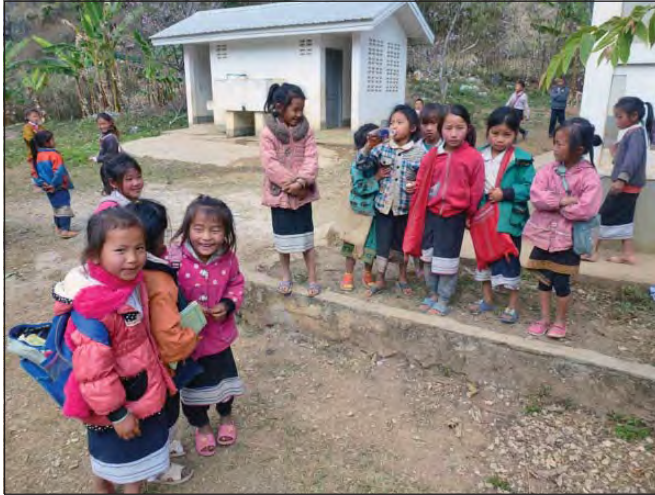
Nasala, where TLCB has funded new tin roofs for two buildings.
