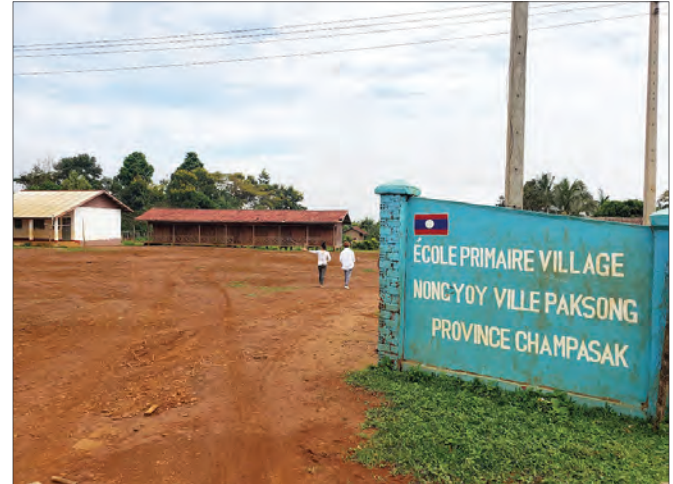
Nong Yoy school in Champassak Province near Attapeu, Laos. The Smiths viewed needed repairs and added it to their list of candidates for future TLCB projects.
