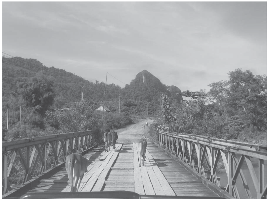
Above, an old US "Bailey Bridge," temporary combat engineer structures that are widely used in Laos and still serving very well. Bottom left, modern roads and bridges are slowly replacing scenes such as the one above. Photos by Mac
