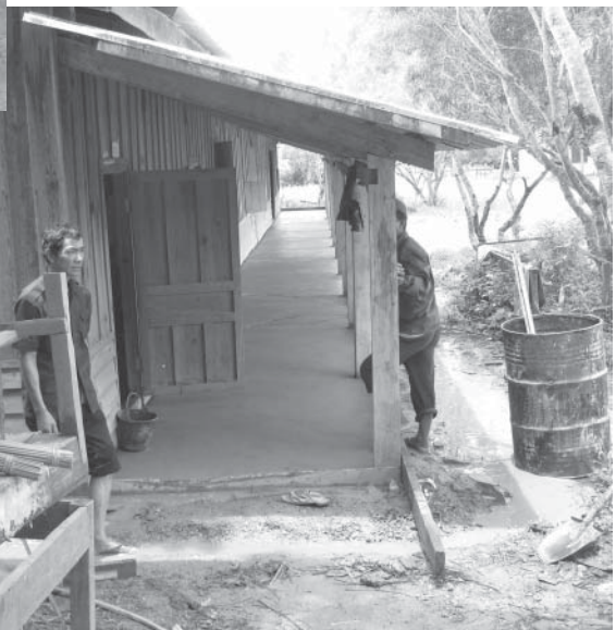
Below, freshly poured concrete porch finishes the Phosy school project. Photos by Mac.
