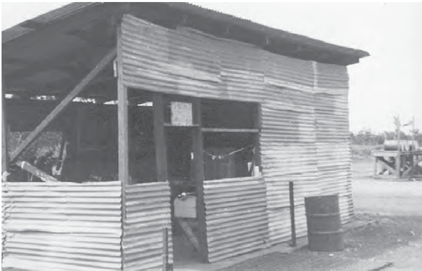
This was the helicopter maintenance workshop at Nakhon Phanom in 1964.
