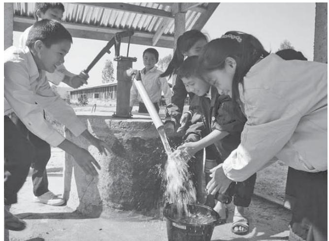
Above, kids show delight with the repaired pump.
