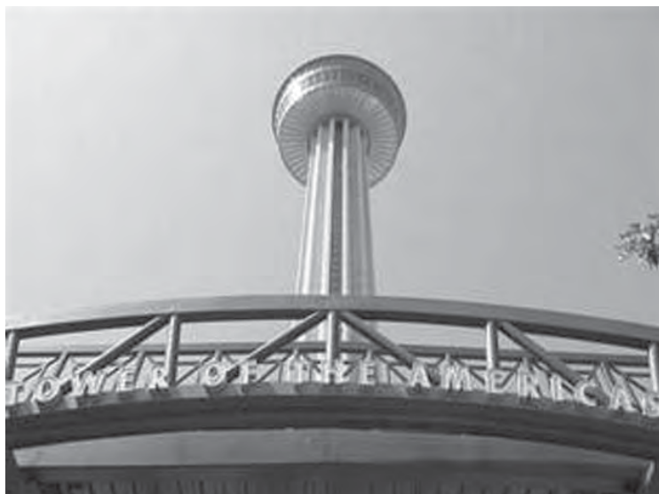
Tower of the Americas, with its rotating restaurant. This is a likely tour site for the Brotherhood.
