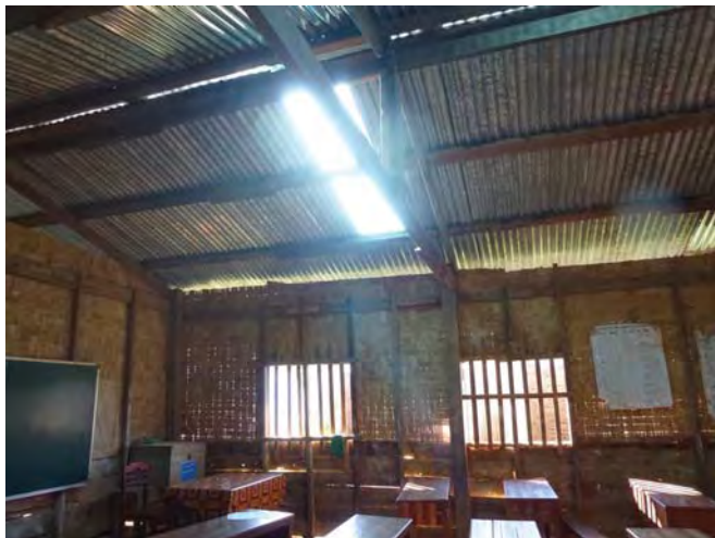
TLC Brotherhood Assistance grant paid for the new roof and the new translucent panels that light up the room. Most schools do not have electricity up here.
