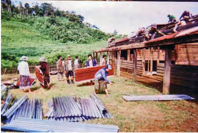
Above, villagers pitch in to instal new school roof. TLCB Assistance provided funding to purchase this currogated steel. Below, good for another ten or so years.
