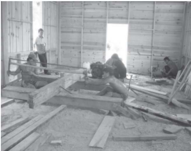
Inside the new dormitory at Pakha—sawing planks the old-fashioned way.
