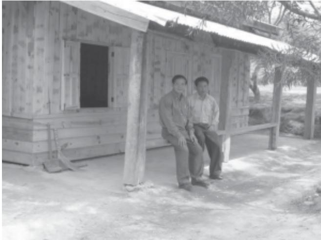
Completed 2008 project—rebuilt life-skills school building ready for school to open at Ban Phosy.
