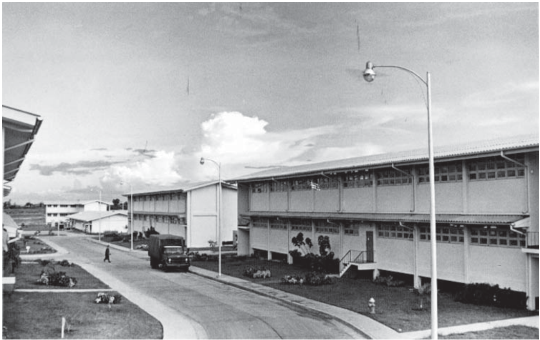
Nothing primitive here! Barracks buildings at Ramasun Station were completed just a few months before Bob Wheatley arrived. "I couldn't believe my eyes," he said, "the place looked like some apartment complex back in the States."
