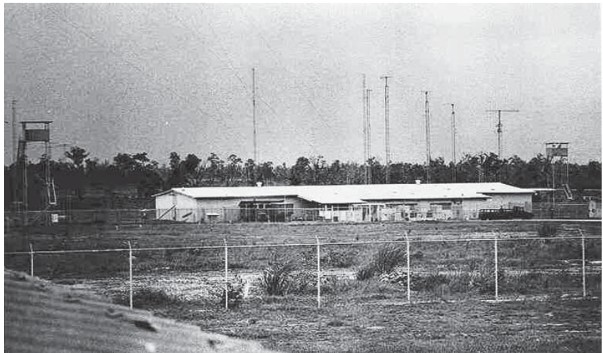
Ramasun secure compound. We can’t tell you any more than that!
