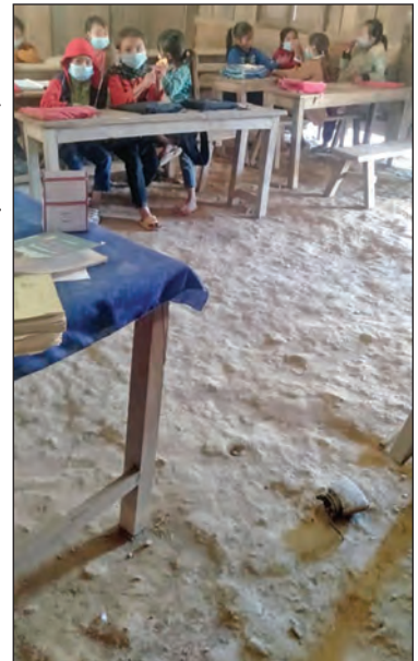
At some schools we have found teachers using the dirt floor as a "blackboard." Having concrete floors will be a real upgrade!, nevertheless!
