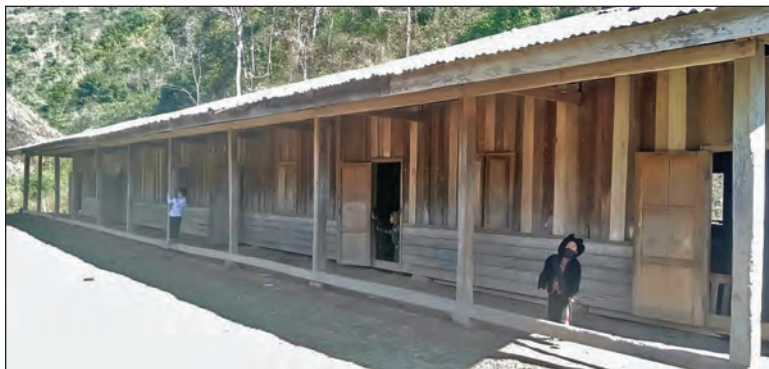
The front of Na Kang Koi Village Primary School, as it looks today.. Photos sent to our SEA team by school officials in Laos. As usual, our team plans to visit after the work is completed, Covid restrictions permitting. Laos has been closed during much of the pandemic.
