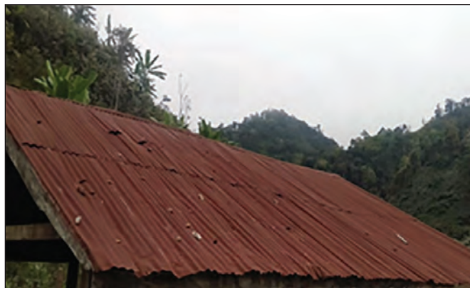
Existing roof. The proposal calls for 420 roofing sheets, 80 pkgs of nails, 6 tons of delivered cement, and 52 cubic yards each of sand and gravel. All labor to be supplied by local villagers.
