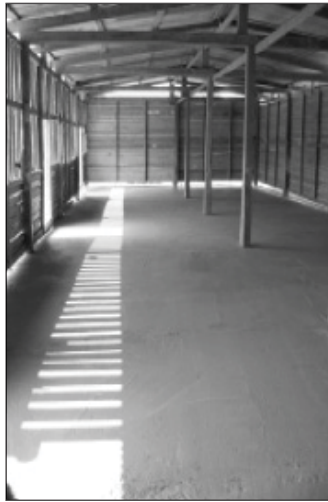
Above, new concrete floor for the Ban Nahom school. Villagers soon picked up the technique and supplied most of the vigorous hand labor. Below, Gome and Jeff pour first bucket of TLCB-donated concrete for the floor.
