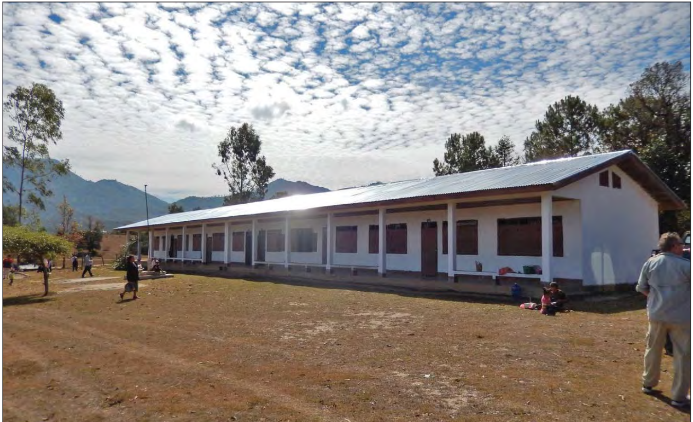
TLCB members can be proud of the shiny new roof on the Ban Boua Thong primary school,
