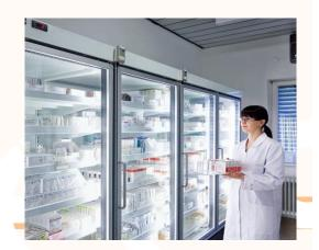
A temperature mapping study is an exercise to qualify temperatures (and humidity if required) of storage environments used for temperature sensitive products. This can include but is not limited to Warehouses (Controlled, uncontrolled, Dedicated or Multi Market), Cold stores/Fridges, Freezers, Containers, Vehicles, Stability Chambers, Incubators
