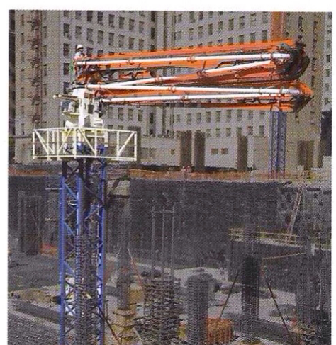
3. Position, pin and pump
