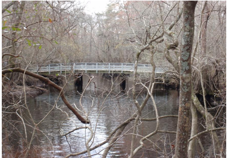
Current Moore's Creek bridge
