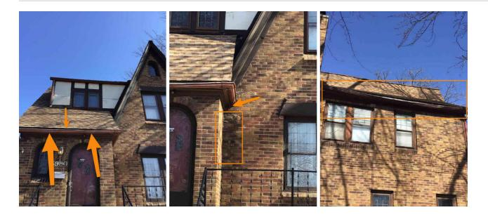
2.2.6 Roof Drainage Systems **DOWNSPOUT DETACHED Downspout is not connected to gutter.**
