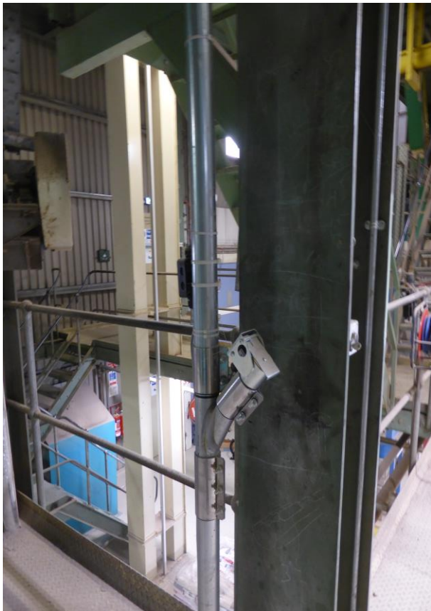
Automatic Valve with Microswitch
