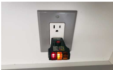
Reversed polarity outlet
