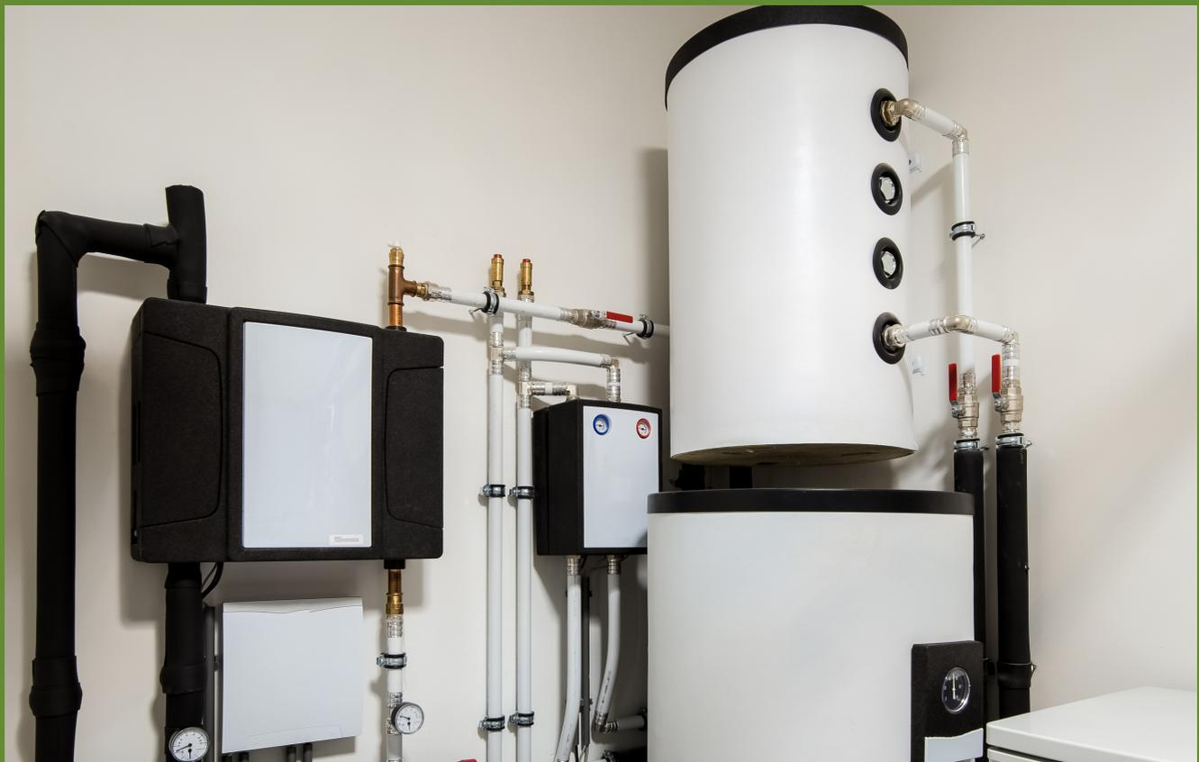
Air source heat pumps are relatively easy to install but lose some of their efficiency during the winter months as the outside air cools down, so auxiliary heating might be needed.
