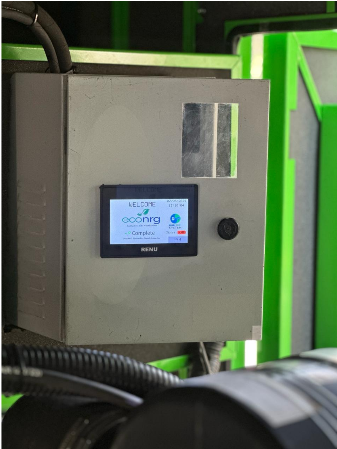
PLC Display with Dedicated Panel for Dual Fuel Controller , Pressure Sensor, Solenoid Valve & Gas Filter
