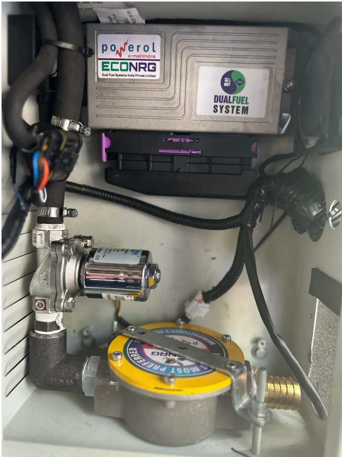
Compact System installed within Dual Fuel Panel and controlled electronically which eliminates any chance of human error.
