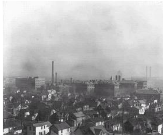
Figure 10: Historic Ancker Hospital
