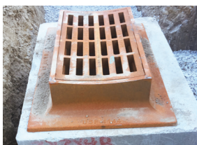
INDOT Contract # B-39578 Lauramie Creek, Superior Construction, Fall 2019
