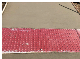
INDOT Contract # R-39327 Asphalt Resurface, Plainfield, IN E & B Paving, Spring 2020
