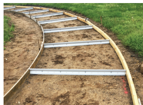
City of South Bend Freemont Sidewalk Project, Walsh & Kelly, Fall 2019
