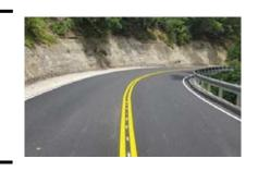
Lewis and Clark Parkway - (Clarksville, IN) - JTL provided survey, design, and specifications for the construction of approx. 8800' of widening, patching and a structural overlay. Former S.R. 131 (renamed Lewis & Clark Park- way) was widened from a rural four-lane road with shoulders to an urban six-lane road with raised medians with landscaping in some sections. Improvements also included curb and gutter, sidewalks, decorative street lighting and landscaping behind the sidewalks on both sides.
