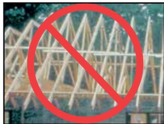
Improper bracing scheme - Continuous TCTLR without Diagonal Bracing
