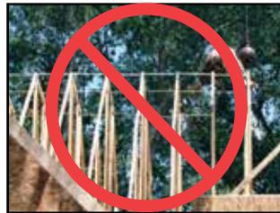
Truss spacers are insufficient as Lateral Restraint and Bracing.
