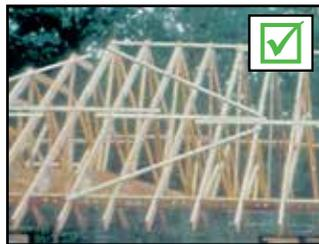
Proper bracing scheme - Continuous TCTLR with Diagonal Bracing.
