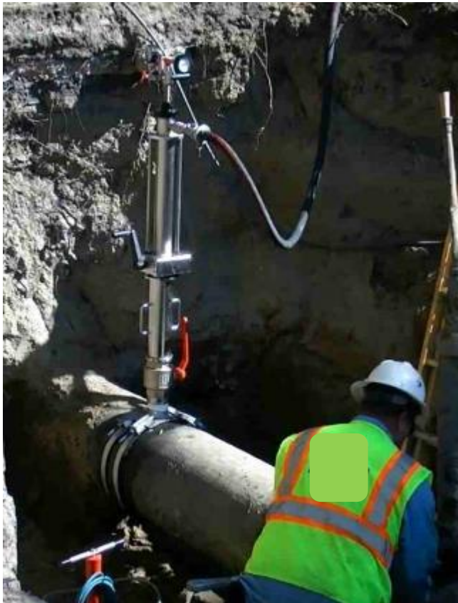
Figure 40. Kleiss stopper installed on the 16” cast iron pipe
