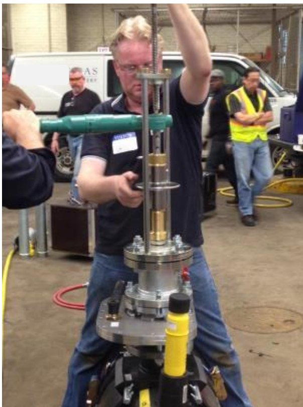
Figure 44. Kleiss BZA-4-G2 tapping equipment – tapping the fitting on the 18” PE pipe
