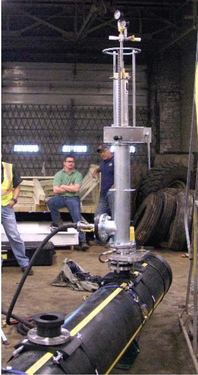
Figure 45. Kleiss stopping equipment on the 18" PE pipe – stopping off 25 psig line pressure
