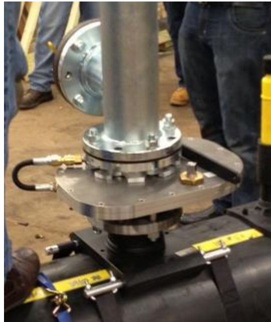
Figure 45. Kleiss stopping equipment on the 18" PE pipe – stopping off 25 psig line pressure
