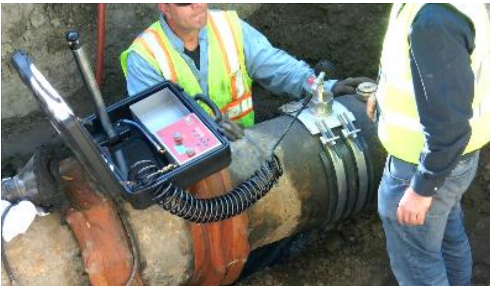
Figure 36. Conducting a pressure test on the fitting prior to tapping
