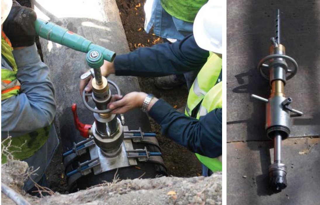
Figure 10. Hot tapping tool for medium and high pressure systems.
