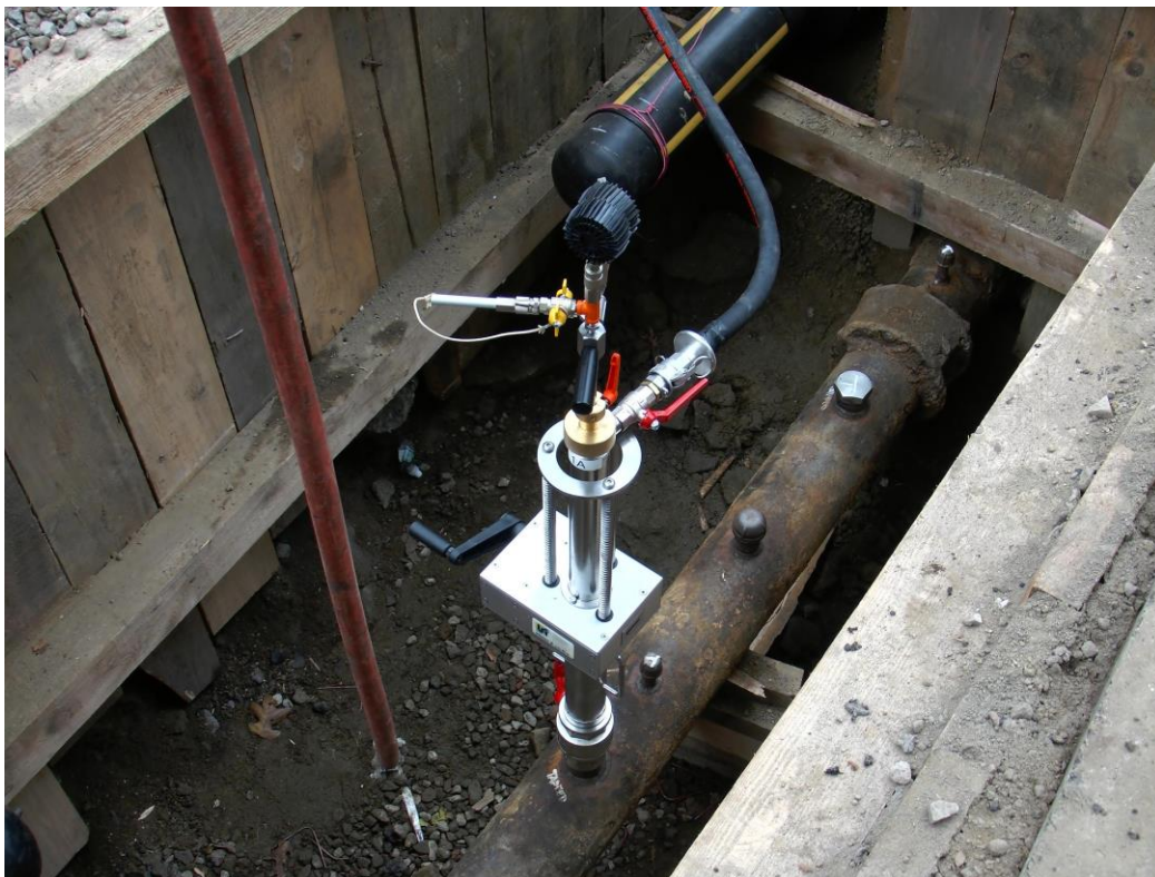
Figure 51. Kleiss BZA-4-G1 stopping equipment installed on the 8” steel pipe
