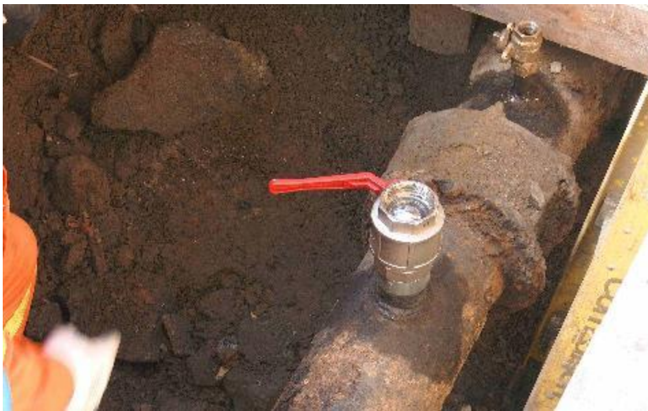
Figure 47. Kleiss weld on fitting and valve installed on the 8" steel pipe
