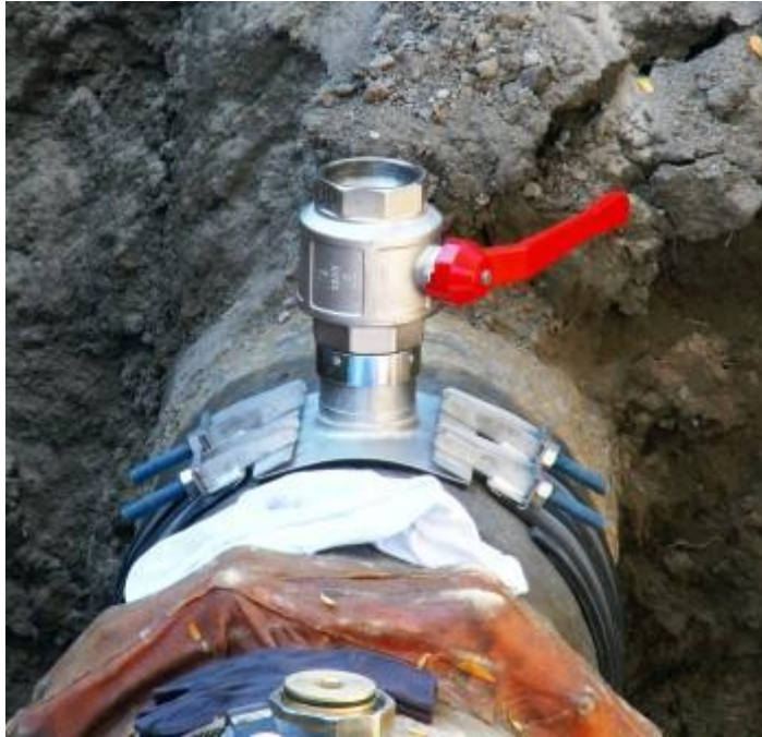
Figure 37. Attach Kleiss saddle and ball valve attached
