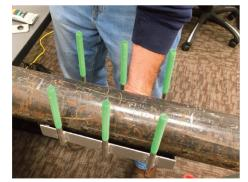
4. Install the lower and upper portions of the fitting onto the pipe. Position the upper half in direct contact with the pipe, the lower half will cradle the upper half. (See image 6.) Make sure the gasket is flat and not wrinkled or folded.
