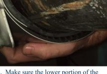
6. Make sure the lower portion of the fitting covers the upper gasket flaps. If there are issues with a tight fit or rolling the gaskets, use a small amount of lubricant on the rubber gasket to reduce friction.
