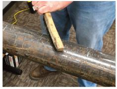
2. Clean (or descale cast iron) pipe of any dirt, debris, or foreign material. Be sure to clean all the way around the pipe and extend the cleaned area slightly outside the size of the fitting.
