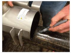
1. Mark the area where the fitting will be installed. Mark both sides and avoid any welded areas.
