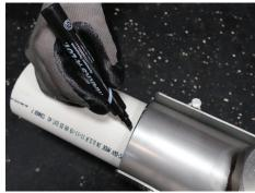
1. Mark the area where the fitting will be installed. Mark both sides and avoid any welded areas.
