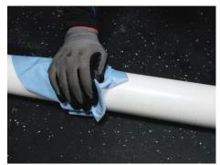
2. Clean pipe of any dirt, debris, or foreign material. Be sure to clean all the way around the pipe and extend the cleaned area slightly outside the size of the fitting.
