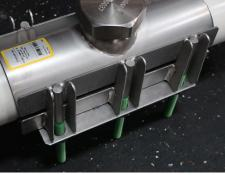
3. Install the lower and upper portions of the fitting onto the pipe. Use spreader plates and on each bolt make certain there is a washer and nut.
