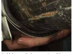
6. Make sure the lower portion of the fitting covers the upper gasket flaps. If there are issues with a tight fit or rolling the gaskets, use a small amount of lubricant on the rubber gasket to reduce friction.
