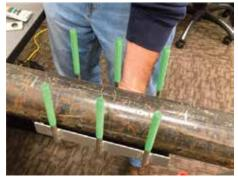
4. Install the lower and upper portions of the fitting onto the pipe. Position the upper half in direct contact with the pipe, the lower half will cradle the upper half. (See image 6.) Make sure the gasket is flat and not wrinkled or folded.
