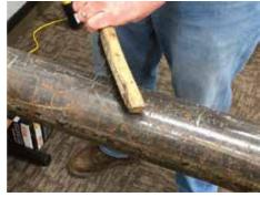
Clean (or descale cast iron) pipe of any dirt, debris, or foreign material.
