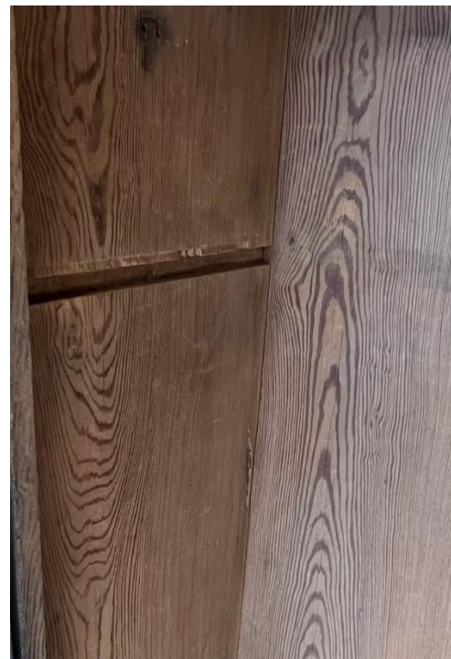
Figure 22: This photo shows the upper dovetail part of the joint ripped out, to the left, enough for the original shelves to slide from the 90-degree base upon their forced removal.
