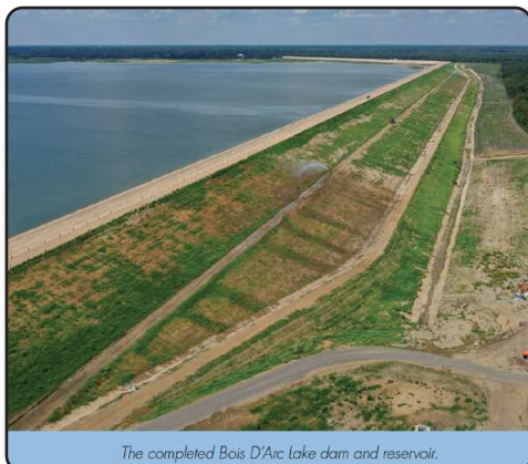
The completed Bois D'Arc Lake dam and reservoir.
