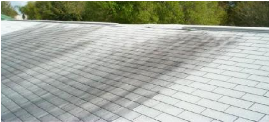
A 5-year-old roof in Florida. The extent of black streaks caused by algae may vary based on climatic conditions.
